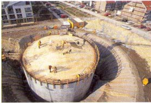
Thermal storage tank under construction
